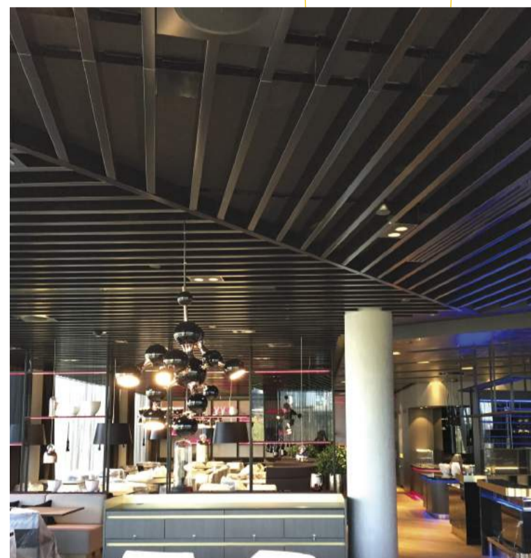
HOTEL HILTON RESTAURANT, TALLIN _ Estonia > vertical baffle 120x40x120 mm
